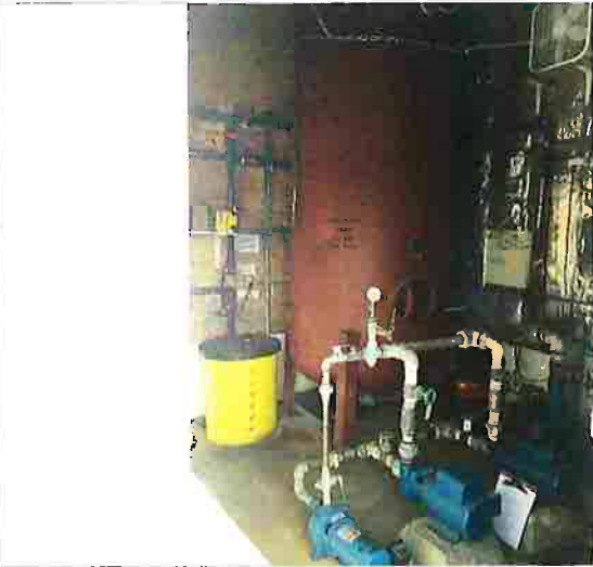
Booster pumps & pressure tank
