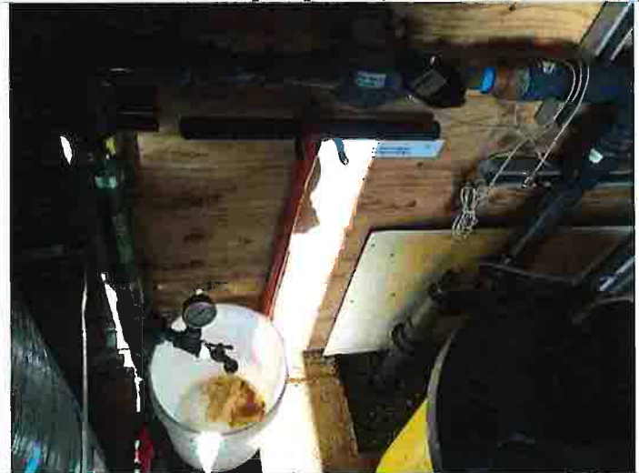
Line from well into pumphouse with KMnO4 injection
