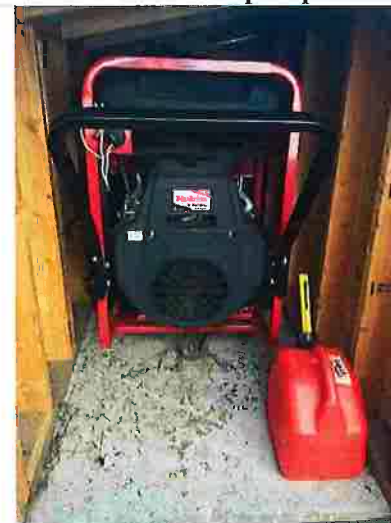
Gasoline powered portable generator
