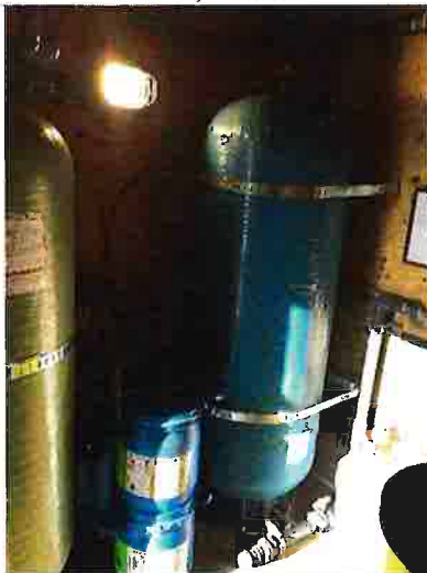
Contact tank (chem feed on the right)
