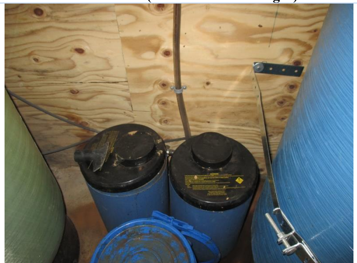
Pot Perm saturators for filter regeneration
