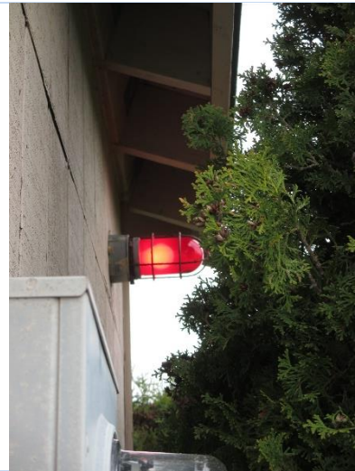
Red light for low reservoir level
