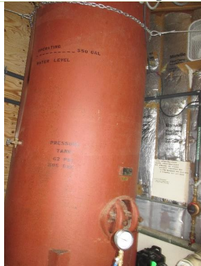
HPN tank, PRV on the back side
