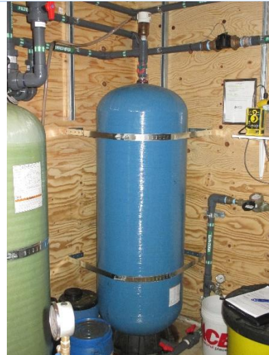
Contact tank (chem feed on the right)
