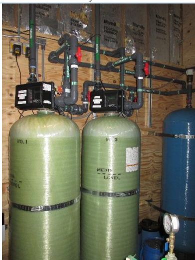
Twin 21" D filters with individual control valves
